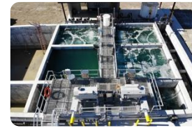
Kyle Texas Wastewater Treatment Plant 150,000 GPD
