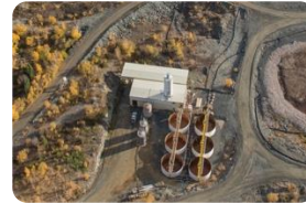
Giant Mine Effluent Treatment Plant 2,750,000 GPD
